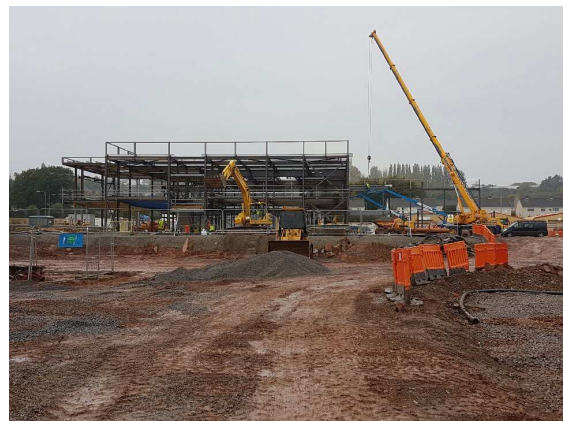
Zone 2, Steel frame
