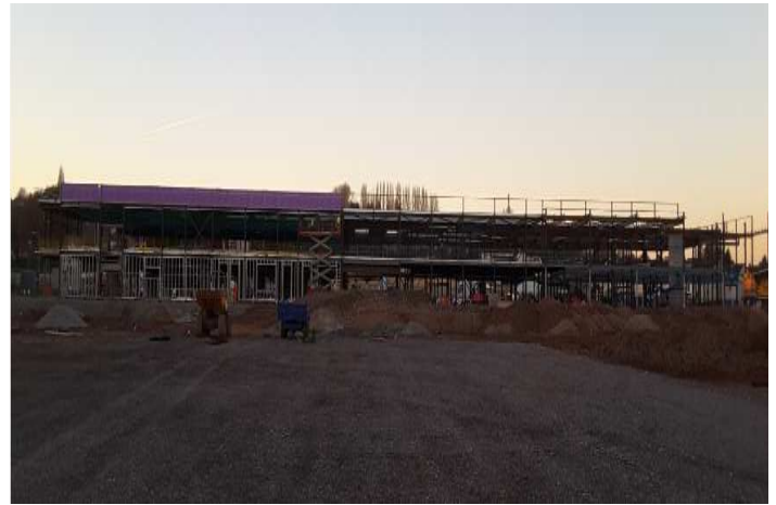
Zone 2, Steel Frame
